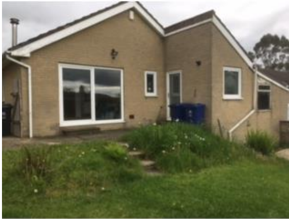
existing rear of the bungalow
